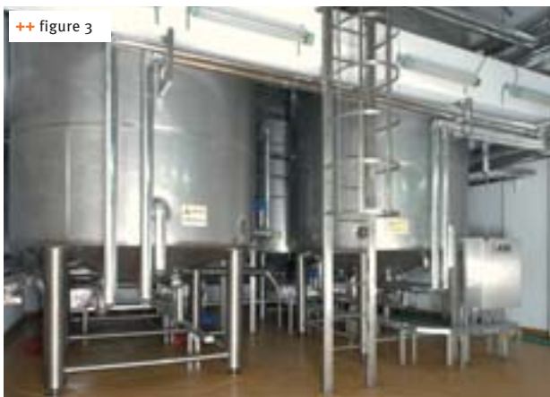
++ figure 3 Oil tanks
